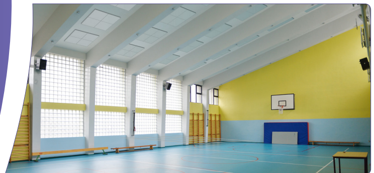
White EcoTech™ panels installed on ceiling
